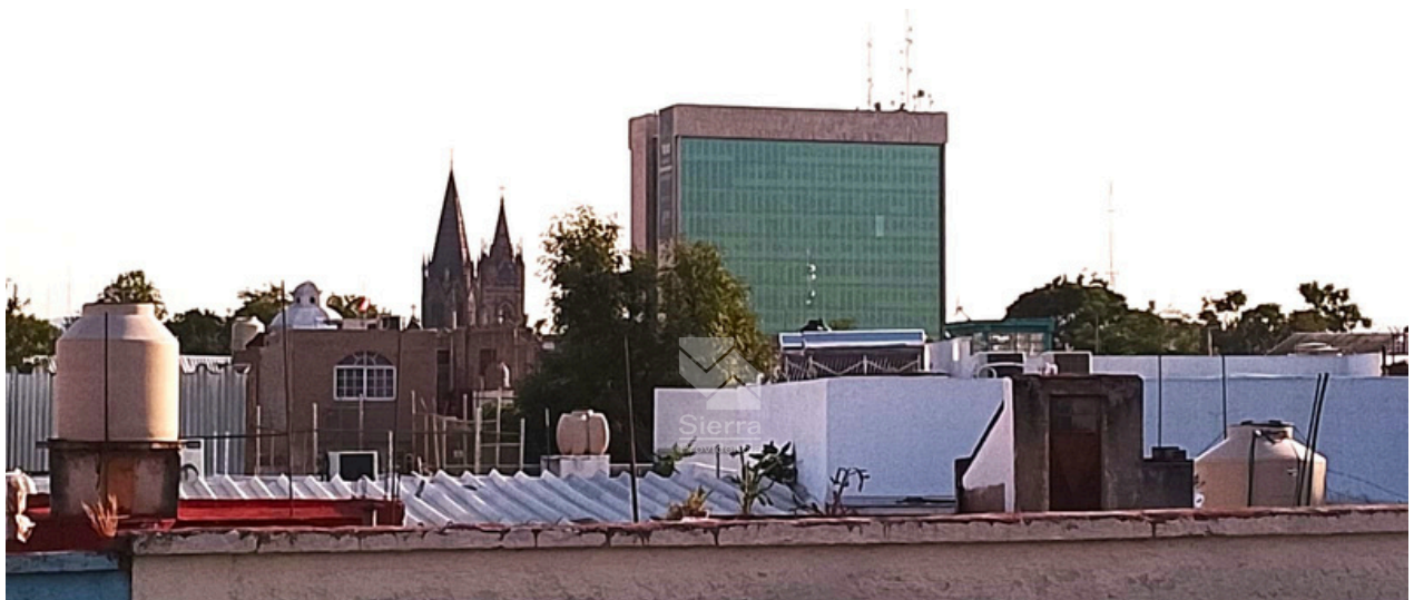
VISTA ROOF TOP
