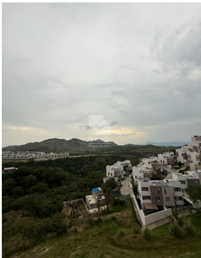
VISTA ROOF GARDEN
