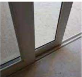
Ventanas de aluminio con cristal claro 6mm y mosquitero | Aluminium windows with a 6mm glass and mosquito screen
