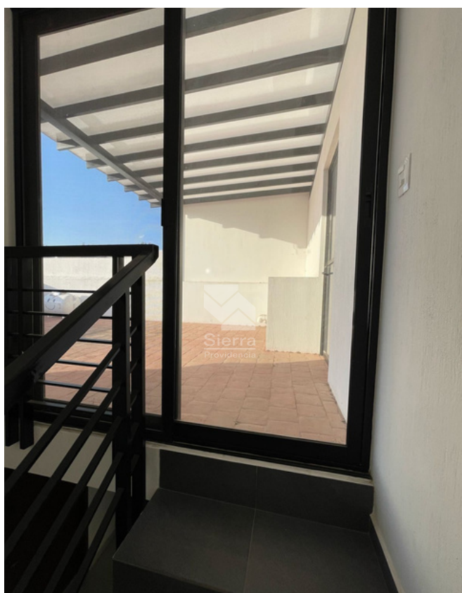
Entrada a roof garden
