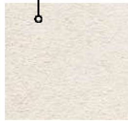
Wall coverings: putty, white stucco White Top Paint
