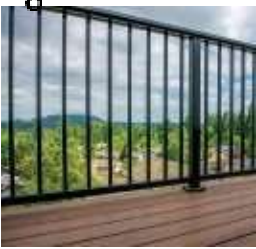
Stair railing, Iron
